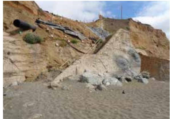
8) Failed sea wall, built without consideration for water erosion
