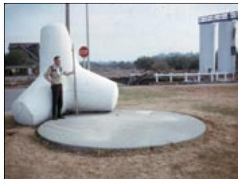
A 25-ton tetrahedron was displaced from a pedestal in Crescent City. Experts calculated the enormous forces required. (A photo taken just after the tsunami showed it was, instead, moved by a huge redwood log pushed ashore in the debris.)
